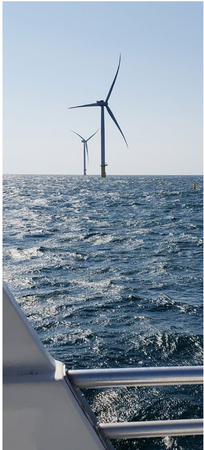
Coastal Virginia Offshore Wind pilot project turbines © Susan Bates
